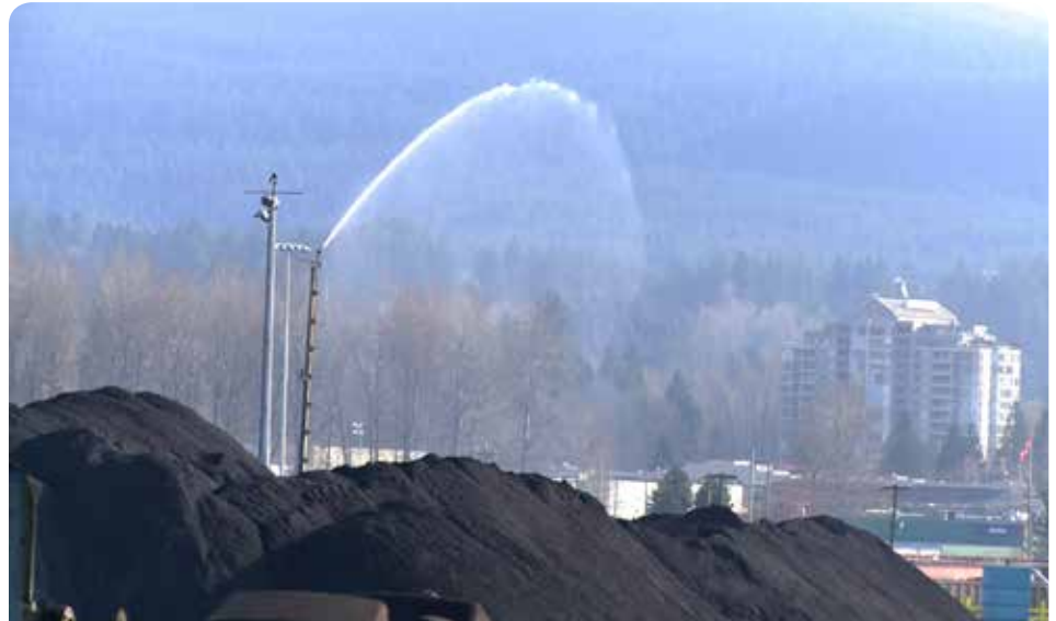
High water spray poles create a water curtain around the coal storage area.
