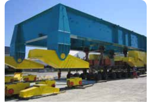
Stacker reclaimer under construction
