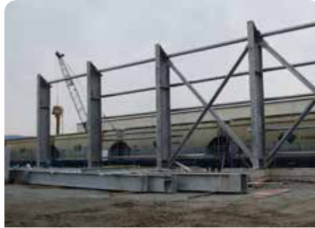
Phosphate rock storage and handling facility under construction
